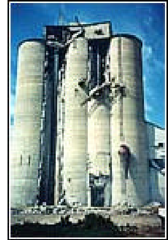
Grain Elevator, Kansas
